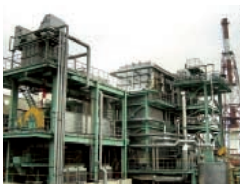
Biomass power generation facilities
