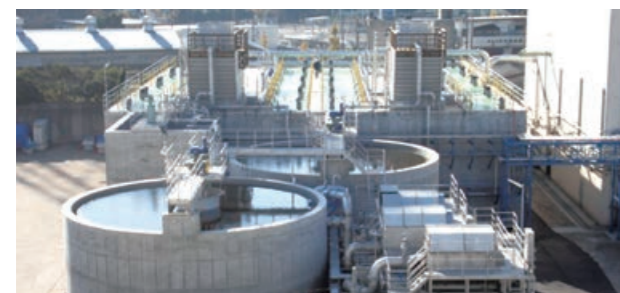
Reused water treatment equipment
