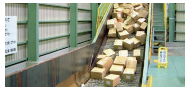
Dedicated equipment for processing confidential paper waste (sample boxes shown in the photo)
