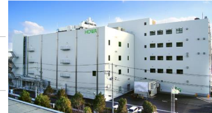
1. New Factory Building, Narashino, Howa Sangyo
