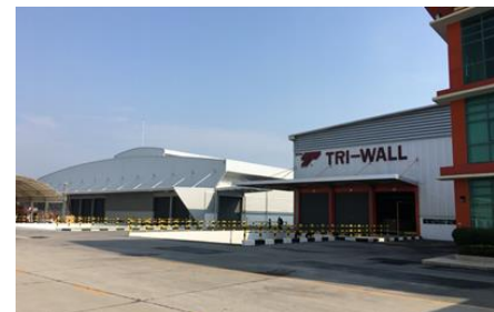
3. The Second Plant, Tri-Wall Packaging (Thai) Ltd.
