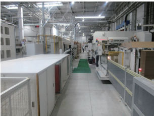
Box making area during renovation
