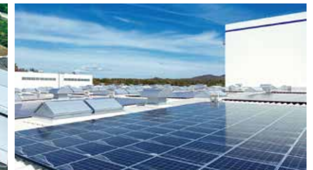
● Photovoltaic panels on the plant building roof
