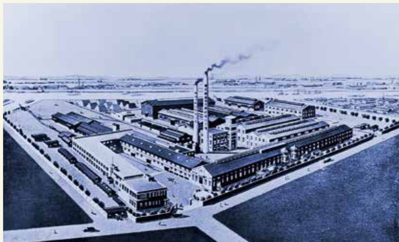
Yodogawa Plant when completed in 1936
