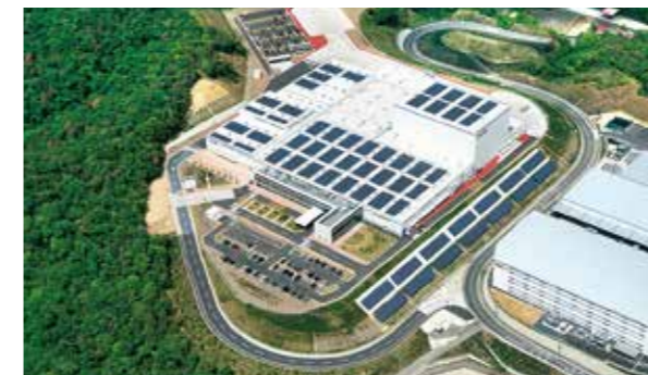
● Bird's-eye view of the Shin-Nagoya Plant
