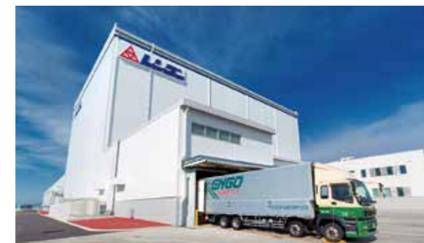
● Rack-type, seismically isolated automated warehouse
