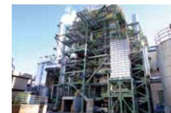
● Wood chip biomass power plant
