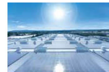
● Photovoltaic power generation system
