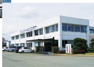
Miyagi Plant (Ishinomaki-shi, Miyagi Prefecture)
