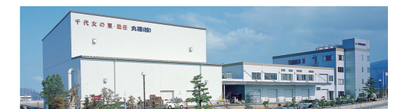
Head Office Plant of Marufuku
