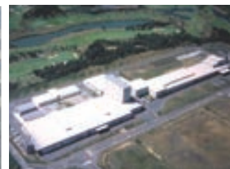
Kanto Plant of Sun-Tox Co., Ltd.
