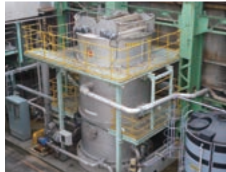
Water treatment system (dissolved air flotation facility)
