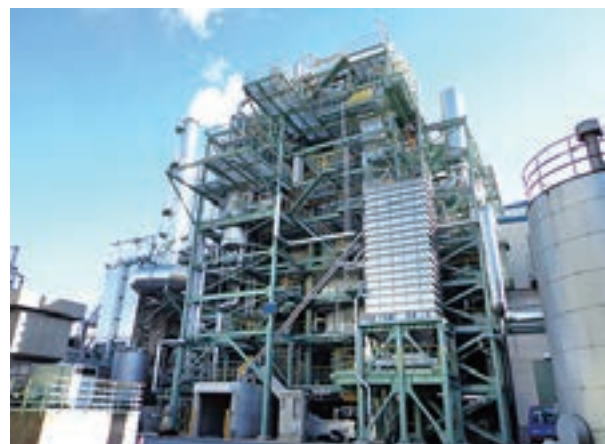
Yashio Mill's wood chip biomass power plant
