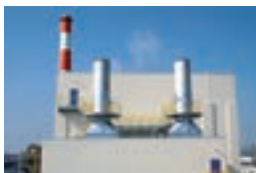
Amagasaki Mill's gas turbine facility
