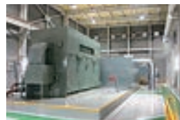
Kanazu Mill's steam turbine power plant
