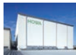
New automated warehouse at Hikata Plant of Howa Sangyo Co., Ltd.
