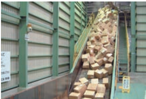
Facilities dedicated to processing confidential paper waste
